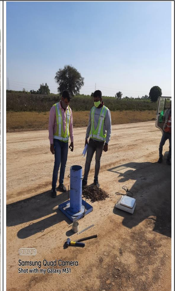
SG top fdd at ch.-360+ 600 to 360+ 720 LHS
