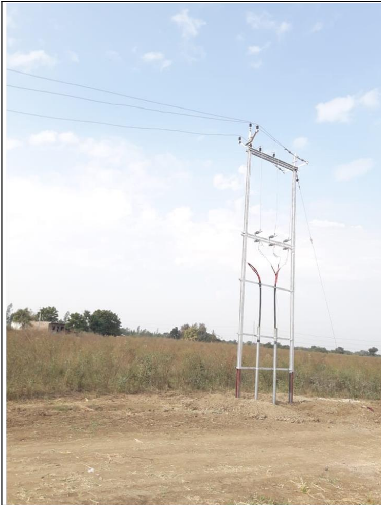
Utility Shifting- Electric line charging at ch.362+650
