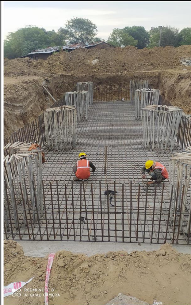
Pile Cap reinforcement binding at MJB 352+281
