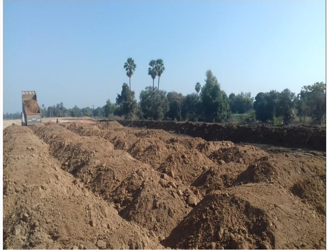
soil dumping In progress at ch.359+230 to 359+450 LHS
