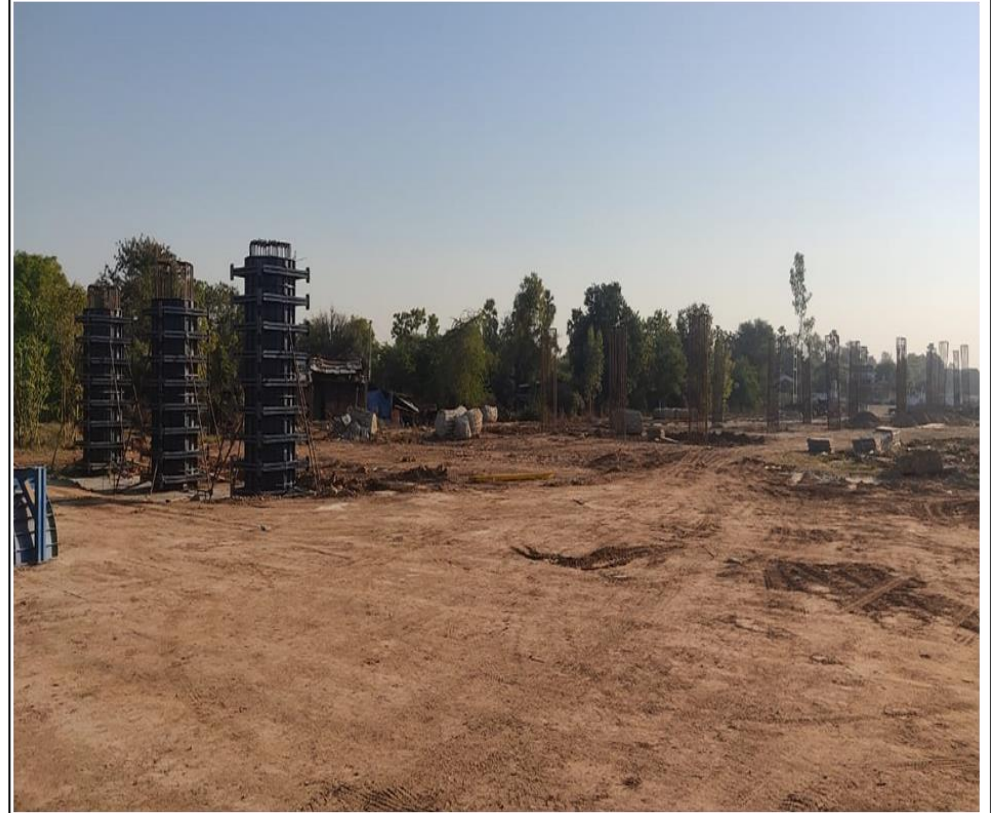
Pier Shaft A1 side LHS MJB @ 352+281
