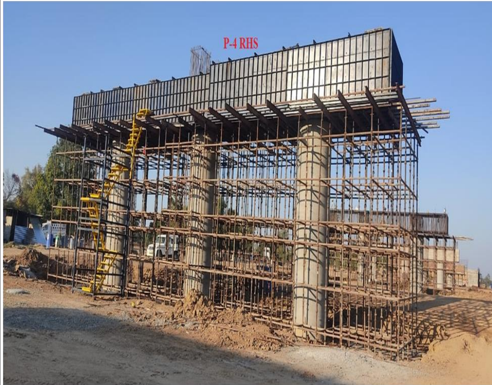
Pier Cap –P-4 RHS A-1 side MJB @ 352+281
