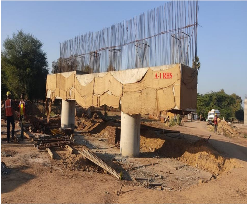
Abutment Cap –A-1 RHS A-1 side MJB @ 352+281
