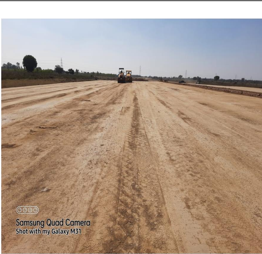
SG top layer rolling in progress at ch 360+600 to 360+720 LHS
