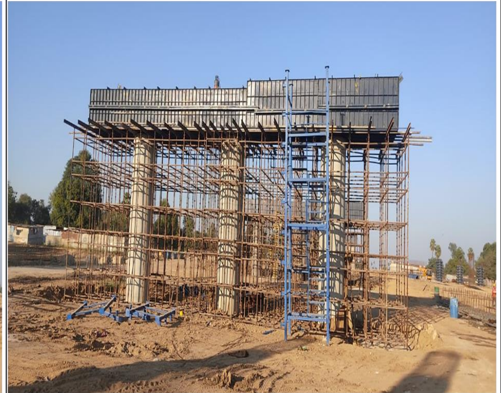
Pier Cap –P-5 RHS A-1 side MJB @ 352+281
